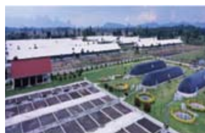
Swine farm with cover lagoon water treatment system
