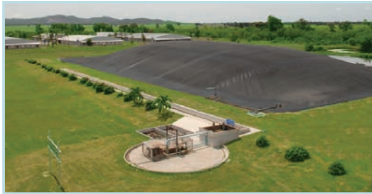
Swine farm with cover lagoon water treatment system
