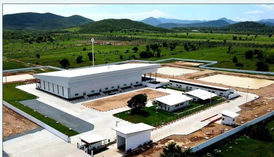
The new state-of-the-art CP food processing factory in Kampot province, Cambodia
